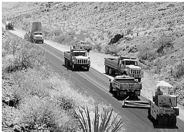
Figure 5—Scrub seal process. (Photo courtesy of Western Emulsion.)
