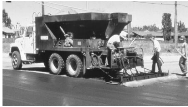
Figure 8—Slurry seal application. (Photo courtesy of Asphalt Institute.)
