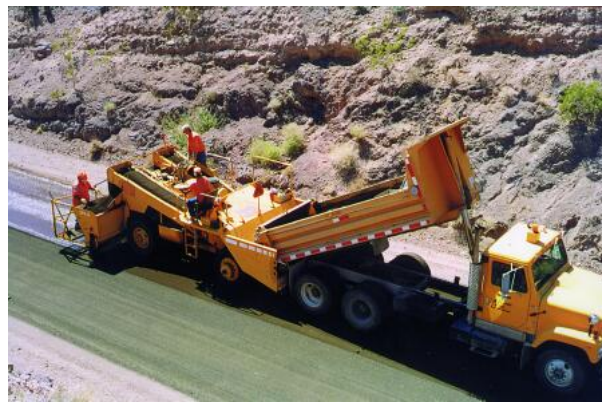
Figure 4—Sand seal. (Photo courtesy of Western Emulsion.)
