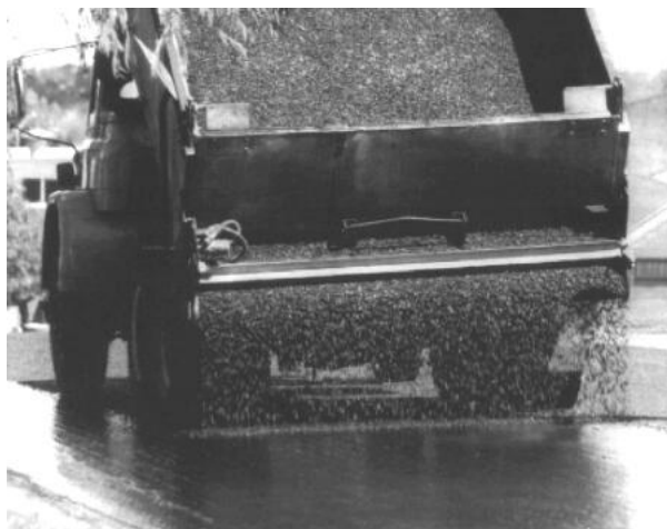
Figure 6—Rock tailgate spreader. (Photo courtesy of Asphalt Institute.)
