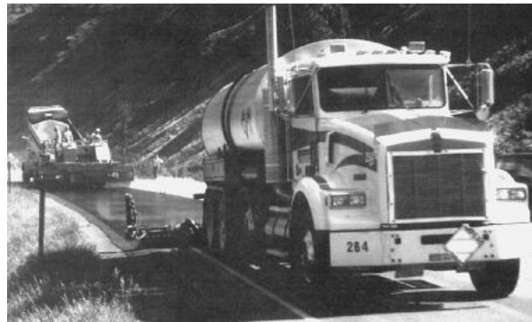
Figure 7—Chip-seal treatment. (Photo courtesy of Asphalt Institute.)
