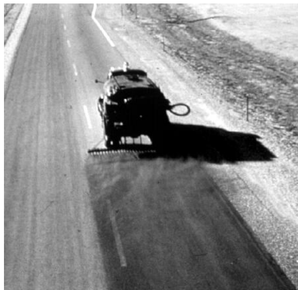
Figure 3—Fog seal. (Photo courtesy of Asphalt Institute.)
